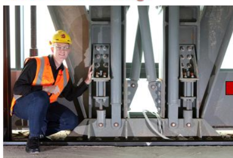
Lead Extrusion Dampers located in key structural locations
